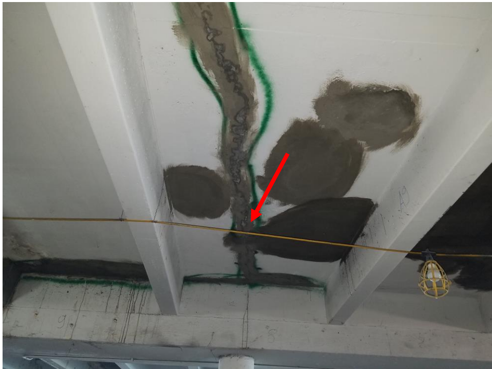
Photo 4: Slab Repair Location where demolition was performed
