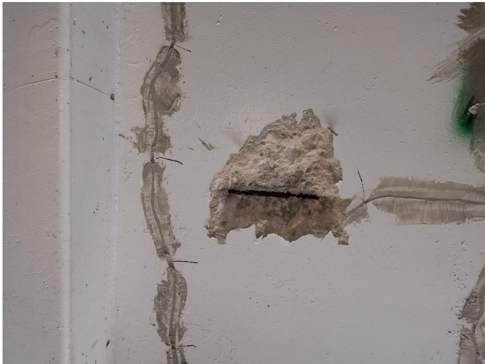
Photo 2: Slab Repair Location where demolition was performed
