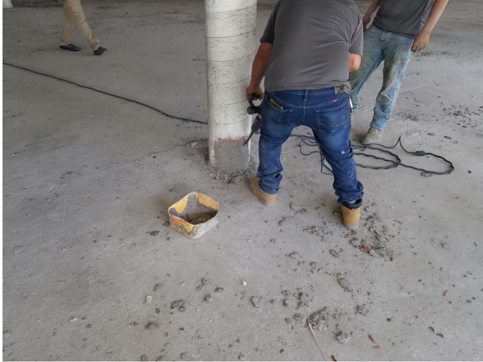
Photo 9: Demolition being performed at the newly repaired column base location
