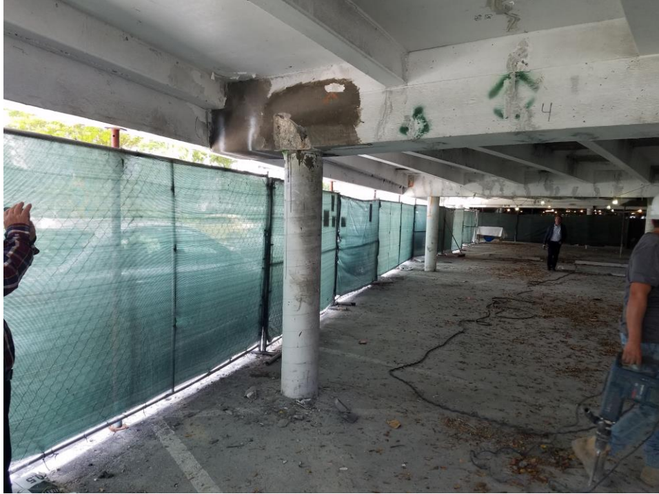
Photo 11: Location of newly repaired beam where demolition was performed
