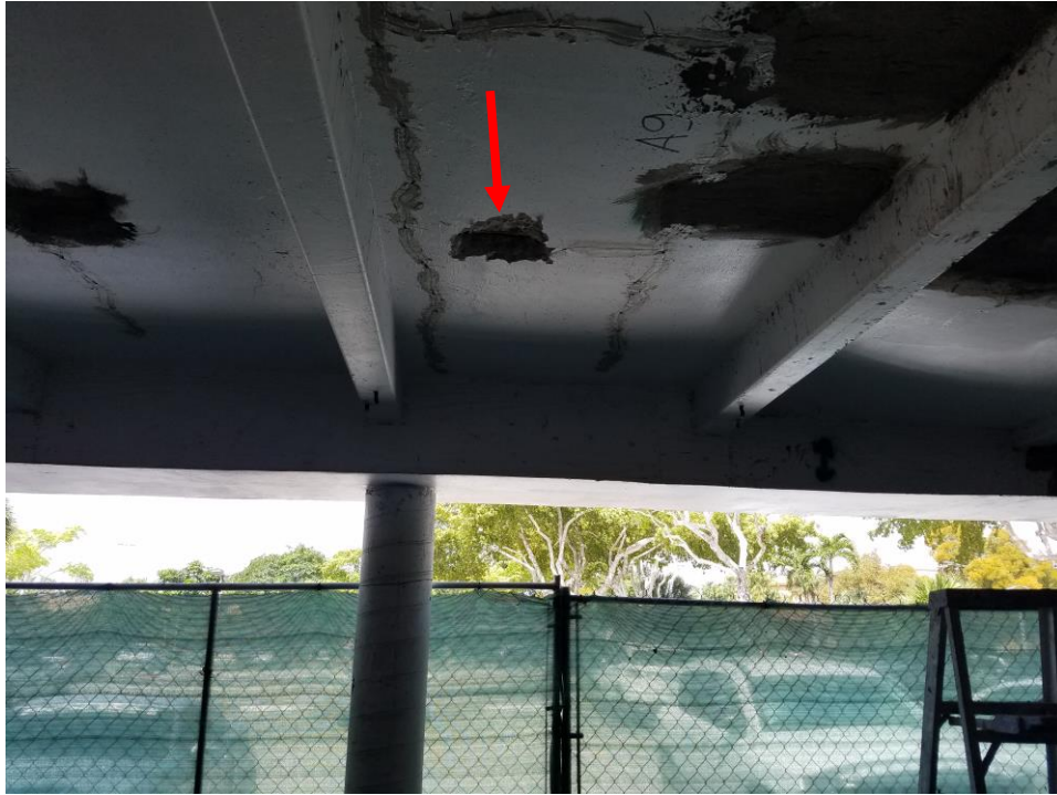
Photo 1: Slab Repair Location where demolition was performed
