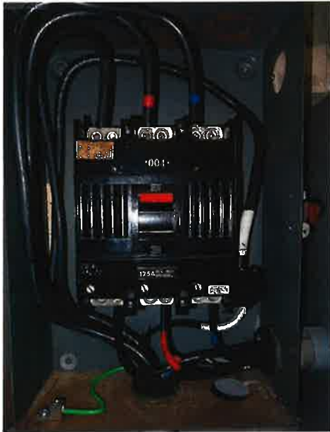
Photo # 121. Wrong color marking for phase conductors (Item # 10-SOUTH-f)
