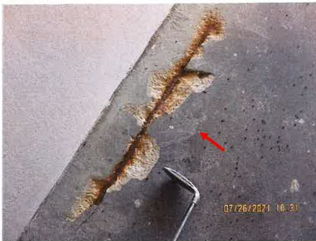
Picture 3: Concrete Spalling and exposed corroded rebar at exterior stairway landing floor.
