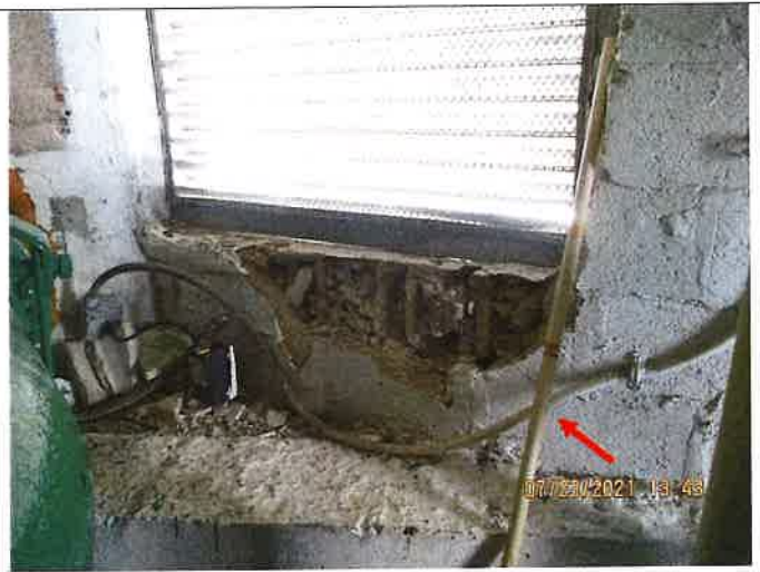
NORTH Roof AHU2
