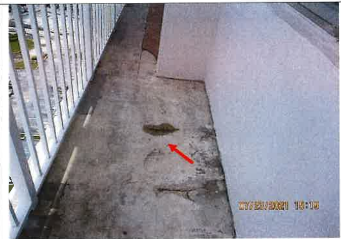
Picture 8: Concrete Spalling and exposed corroded rebar at exterior catwalk / crossover floor.
