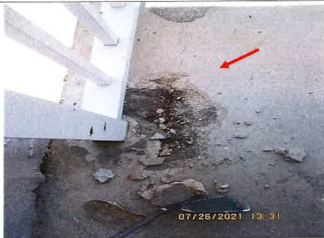
Picture 7: Concrete Spalling and exposed corroded rebar at exterior stairway landing floor.
