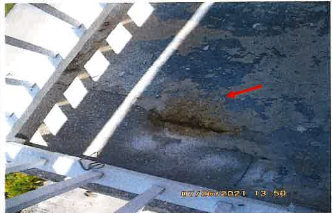
Picture 6: Concrete Spalling and exposed corroded rebar at exterior stairway landing floor.
