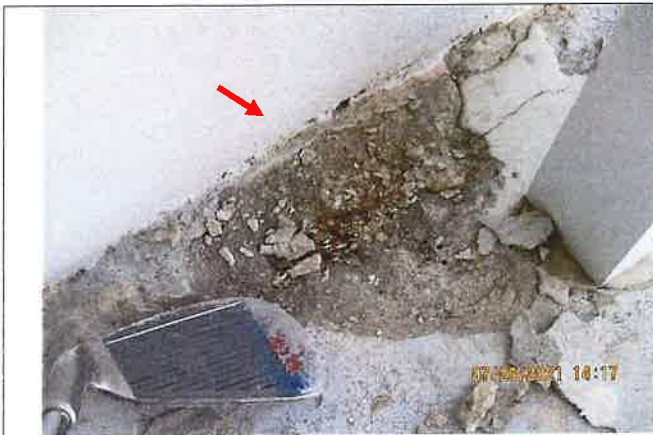
Picture 5: Concrete Spalling and exposed corroded rebar at exterior stairway landing floor.
