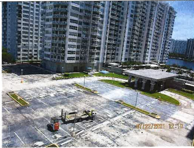
Picture 31 Plaza Del Prado West Deck and Garage not in use.
