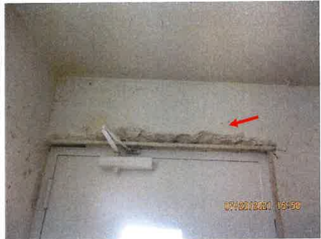
Picture 2: Concrete Spalling and exposed rebar at exterior stairway door header.
