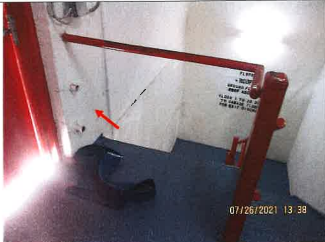
Picture 15: Missing stairway guardrail.
