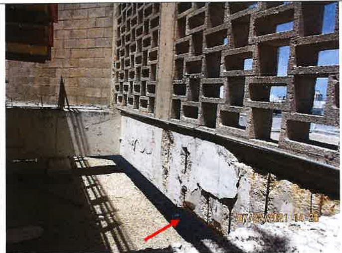
Picture 26: Concrete spalling, exposed corroded rebar at cooling tower enclosure beam supports.
