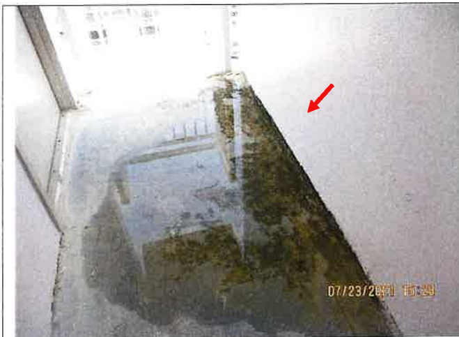
Picture 9: Ponding water and biological growth observed at exterior stairway landing floor.
