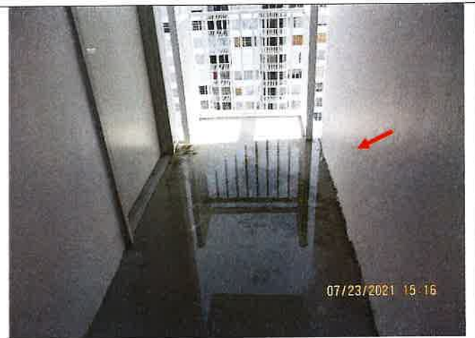
Picture 10: Ponding water and biological growth observed at exterior stairway landing floor.
