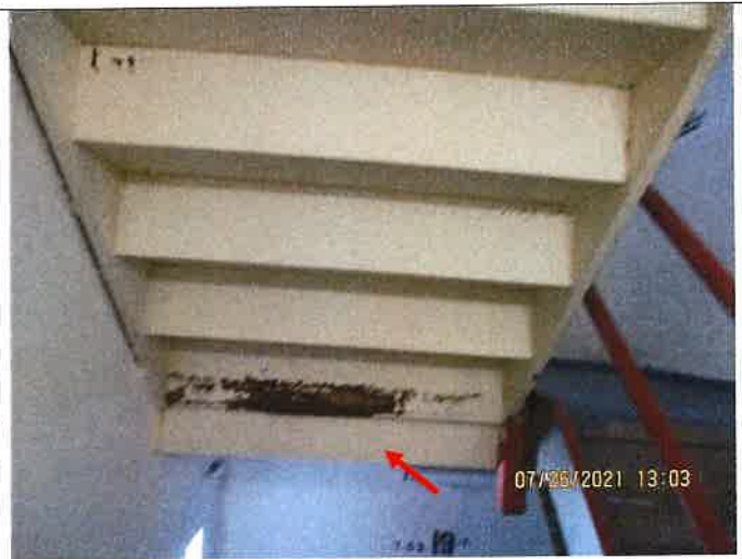
Picture 14: Severely corroded Steel stairway thread and riser condition.
