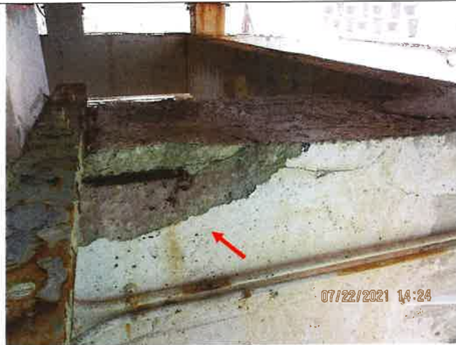
Picture 23: Concrete spalling, exposed corroded rebar at cooling tower enclosure beam supports.
