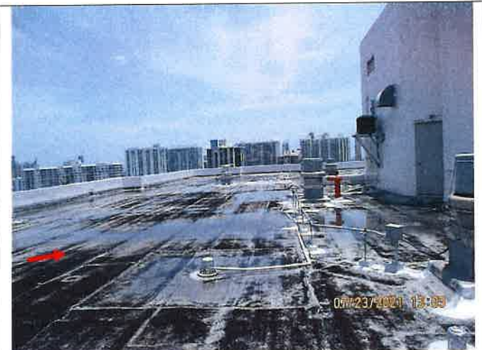
Picture 16: Ponding water and bubbling / blister observed at roof.
