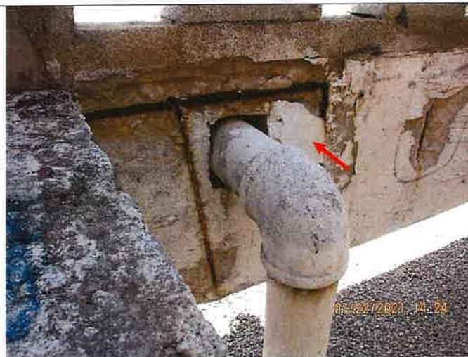
Picture 25: Concrete spalling, exposed corroded rebar at cooling tower enclosure beam supports.
