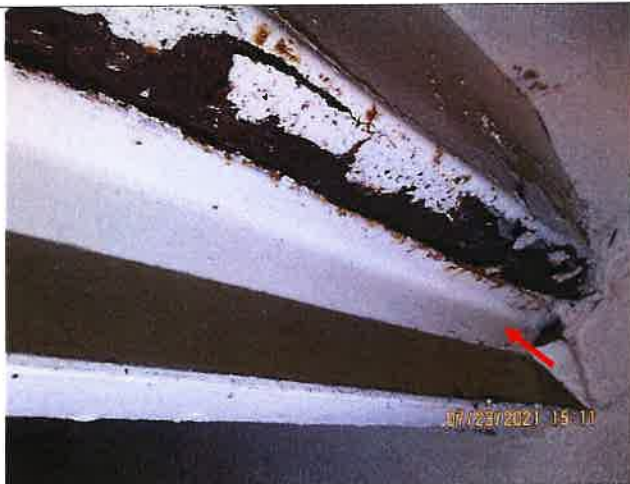
Picture 11: Severely corroded Steel stairway thread and riser condition.
