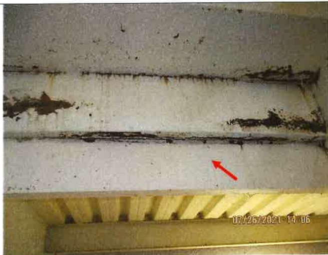
Picture 13: Severely corroded Steel stairway thread and riser condition.
