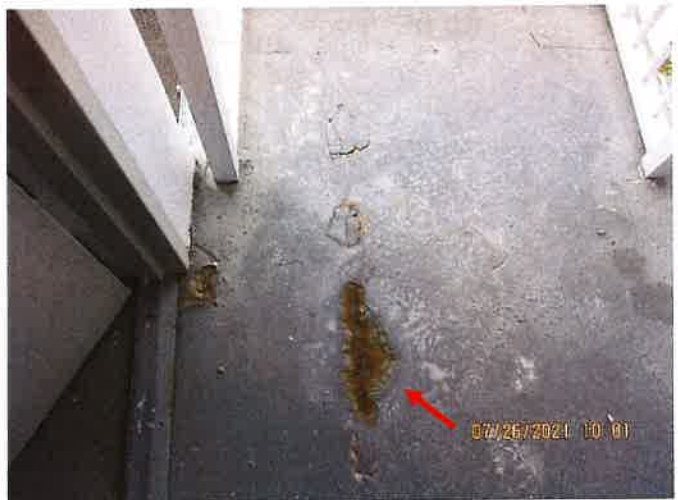
Picture 4: Concrete Spalling and exposed corroded rebar at exterior stairway landing floor.
