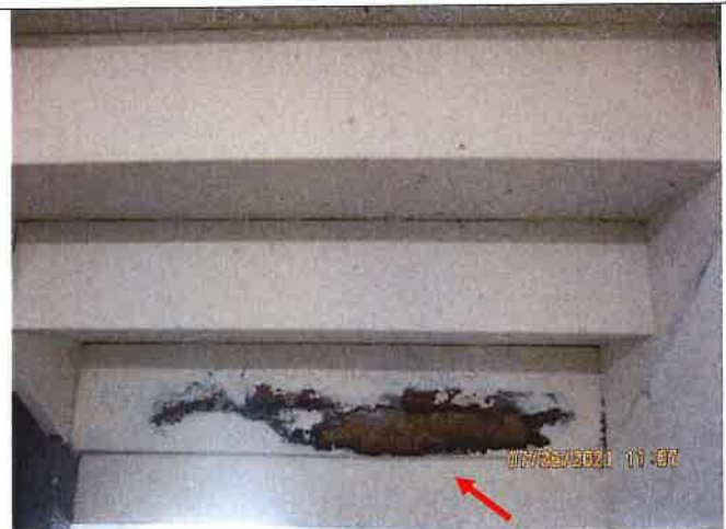
Picture 12: Severely corroded Steel stairway thread and riser condition.
