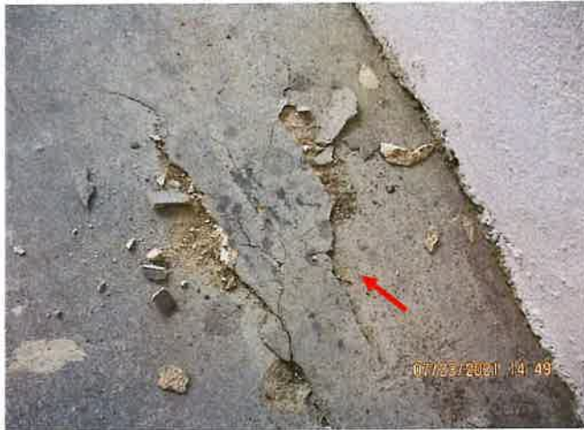
Picture 1: Typical Concrete Spalling Stairway Landing.
