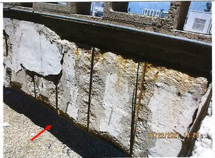
Picture 24: Concrete spalling, exposed corroded rebar at cooling tower enclosure beam supports.
