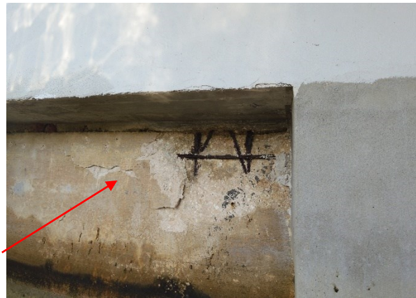
Image 3: Concrete wall panel repair
