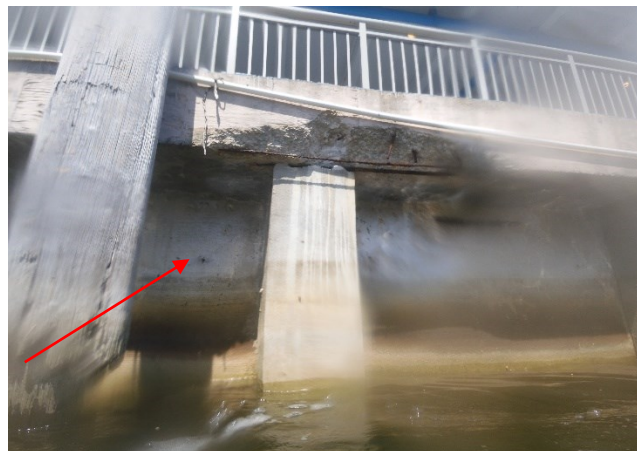
Image 2: Seawall Concrete cap repair
