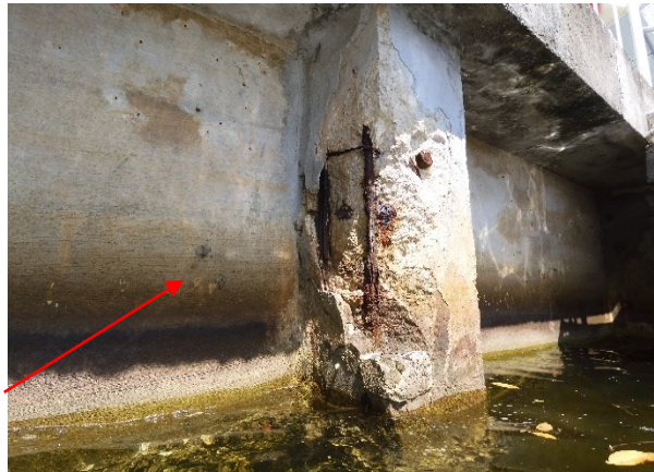
Image 1: Seawall king pile repair
