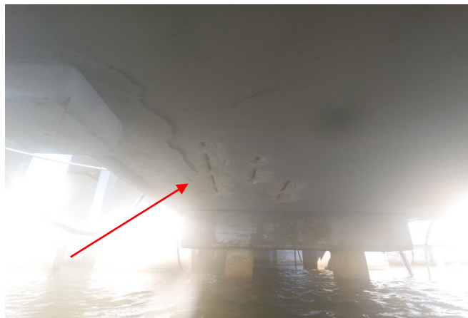
Image 6: Concrete dock floor underside
