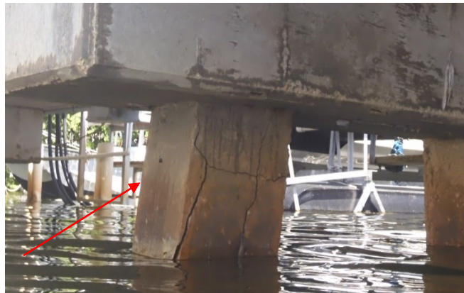
Image 4: Concrete dock pier footing
