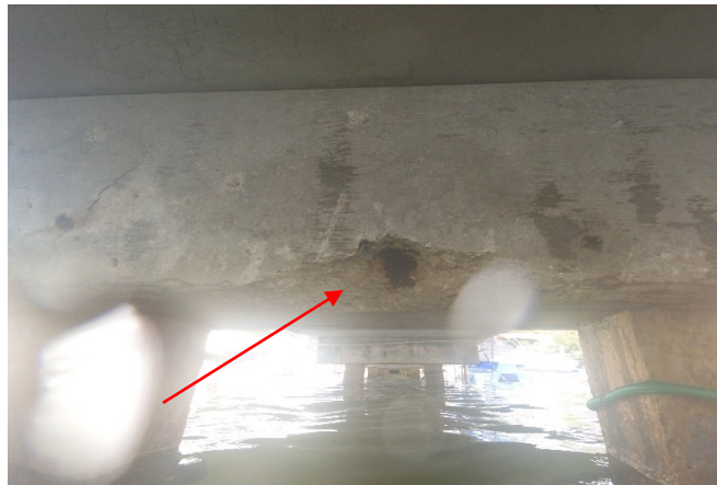
Image 5: Concrete dock tie beam
