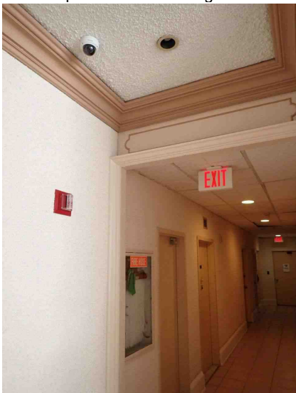
fire alarm pull station, fire hose, security cameras
